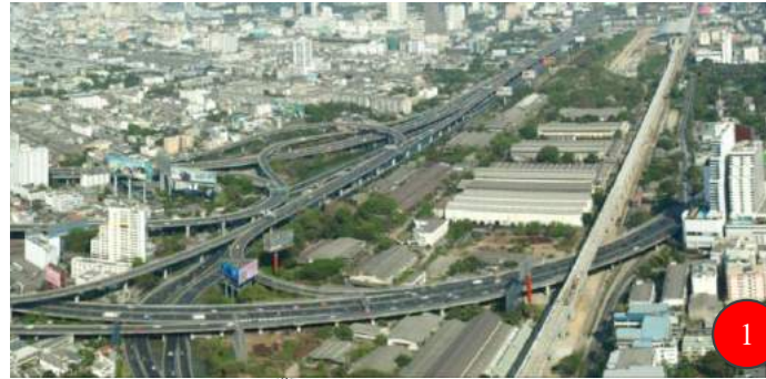
Road within the Site And around the area
